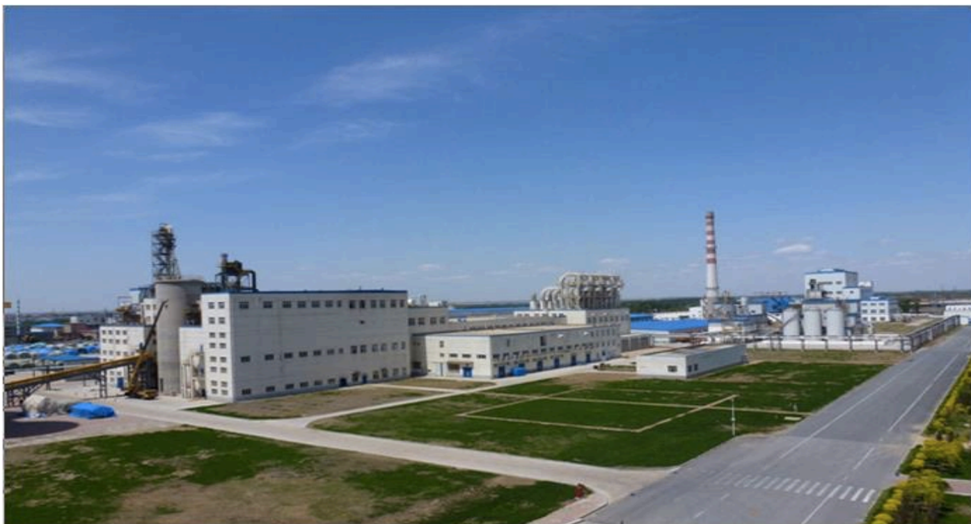
Photo 2 Liaoning Yihai Kerry Starch Technology Co., Ltd Location
